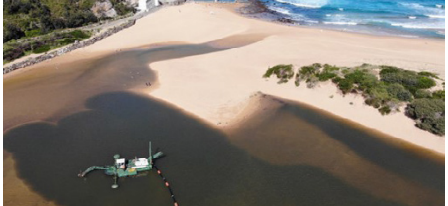
Dredge in entrance of Narrabeen Lagoon in 2021
