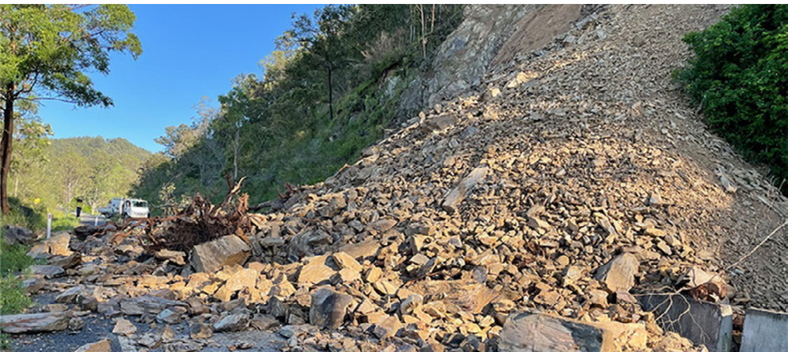
Landslip on Armidale Road, Devil's Nook. Source: Kempsey Shire Council
