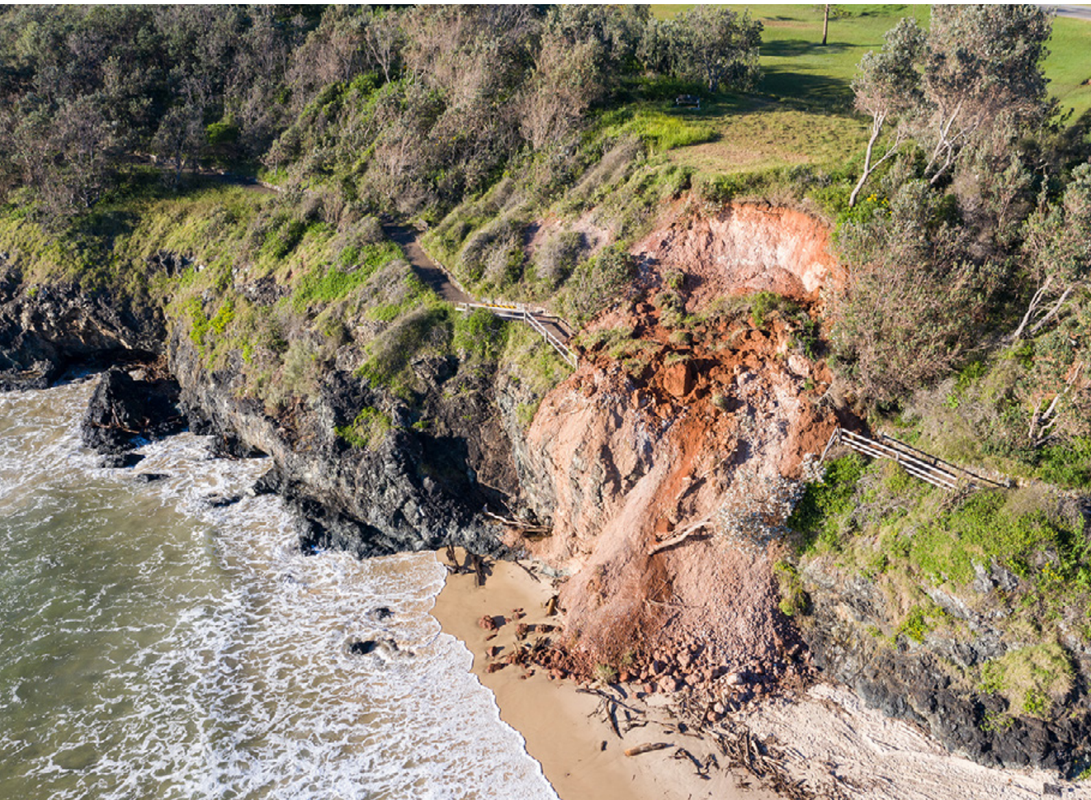
Landslide at Oxley Beach, Port Macquarie
