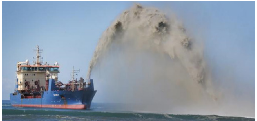
Dredge pumping sand from offshore into the active beach zone 14
